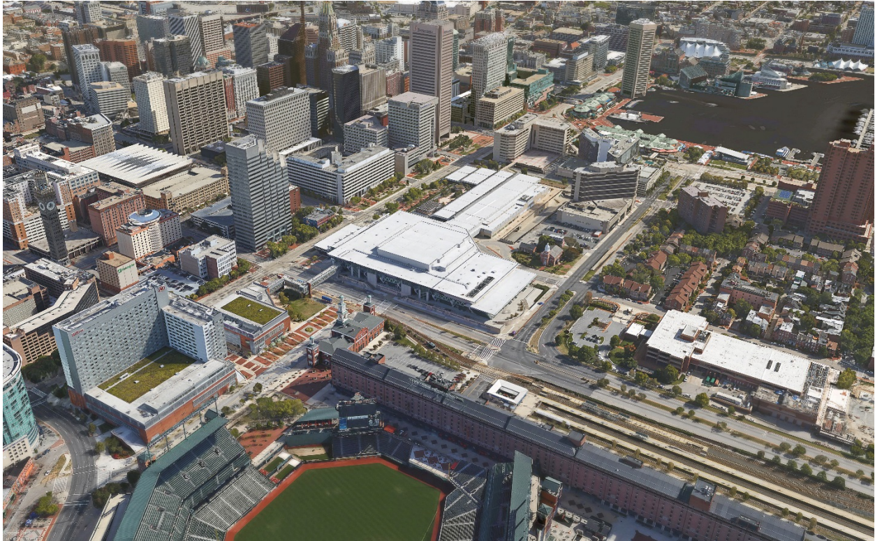
Aerial view of the existing Baltimore Convention Center and study site
